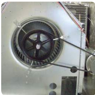
PowerMax DriveN Pulley on a Centrifugal Fan.
