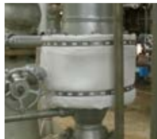
Valve with and without the installed FIRESAFE Fire Protector.
